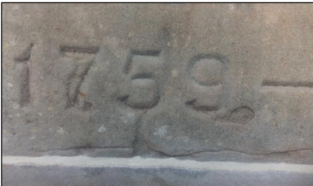
Cracks below the date inscription of before (left) and after (right) Paraloid B72 repair
