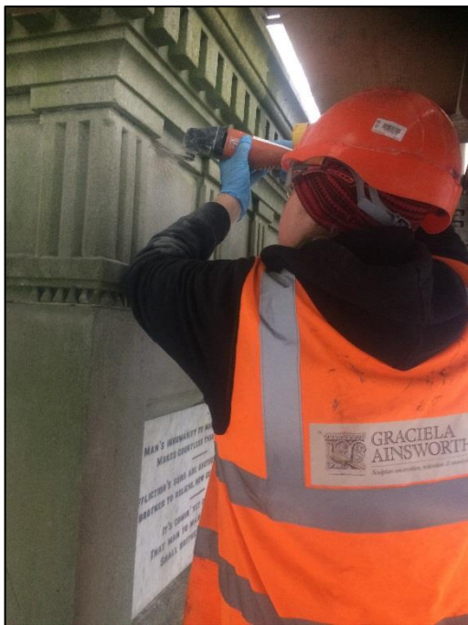
Above: Raking out failed mortar with an oscillating tool
