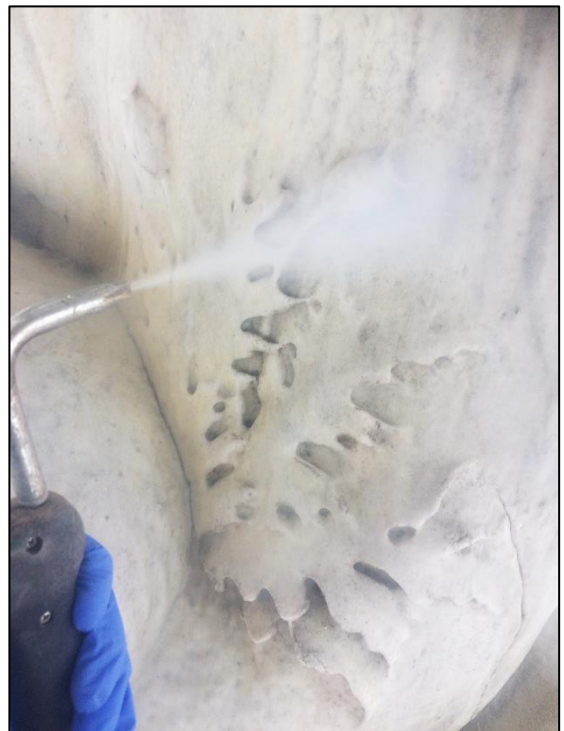
Left: Brush cleaning with water and D/2 biocide Right: Rinsing with clean water
