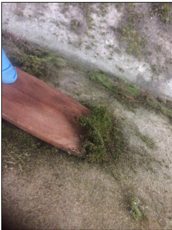
Left: removing moss with wooden tools Right: Steam cleaning more stubborn dirt deposits
