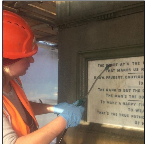
Left: Brush cleaning with water and D/2 biocide Right: Rinsing with clean water
