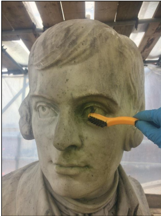
Left: Brush cleaning with water and D/2 biocide Right: Rinsing with clean water
