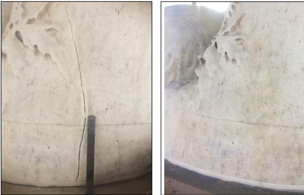
Cracks in the fly plaid before (left) and after (right) Paraloid B72 repair
